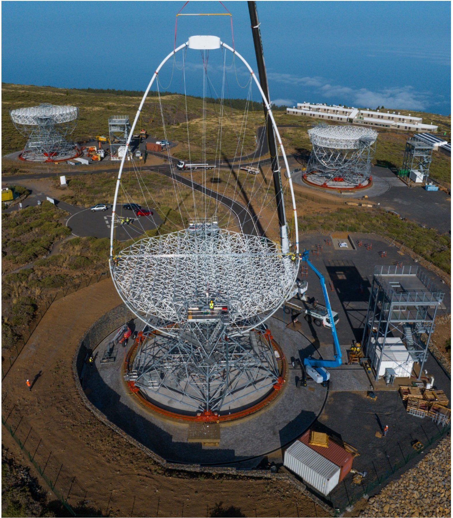
Camera Support Structure installed
