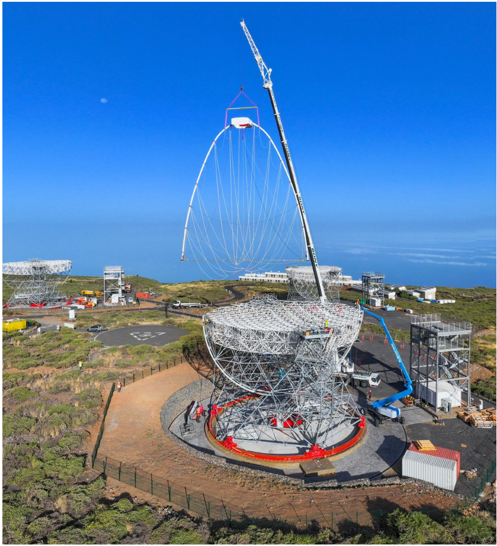
Lifting of Camera Support Structure
