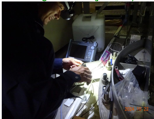
Cutting the fiber (jacket?)
