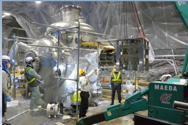
Cryo-cooler unit installation
