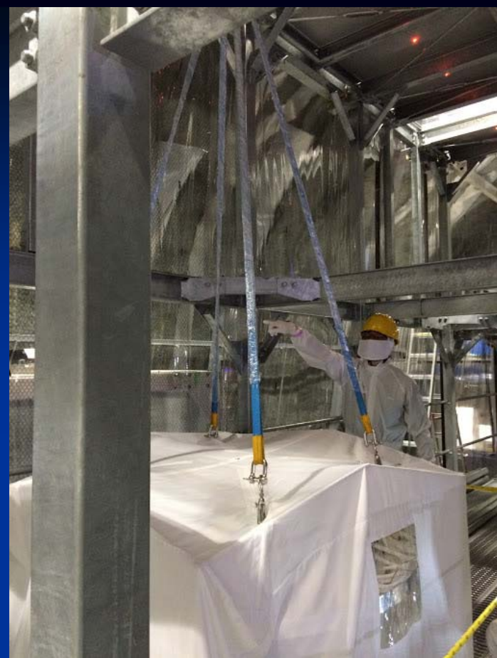
Lift up of suspensions covered by clean bag from assembly frame
