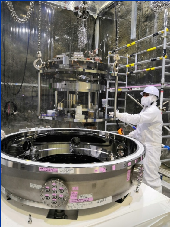
Installation of BF with DP
