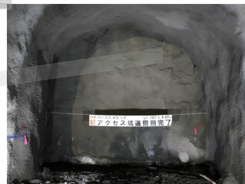
Access tunnel excavation was completed. (2022 Feb.)
