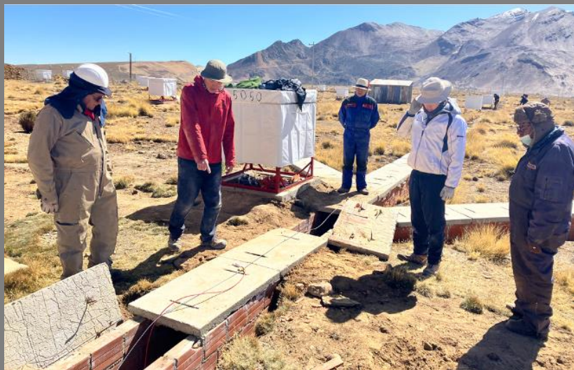
Installation of cables
