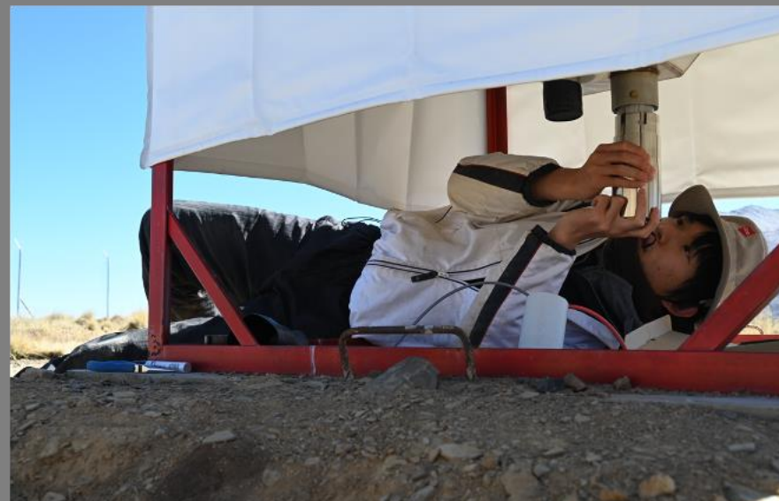
Installation of PMTs
